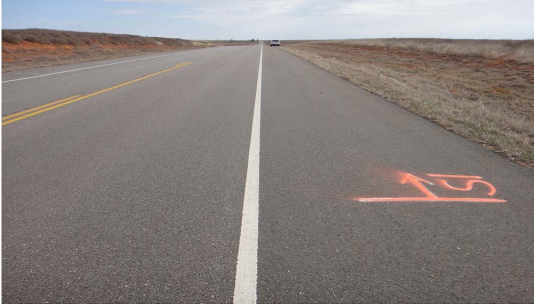
(a) Section 1: RAP/RAS Mix with PG64-34 - No Transverse Cracking.
