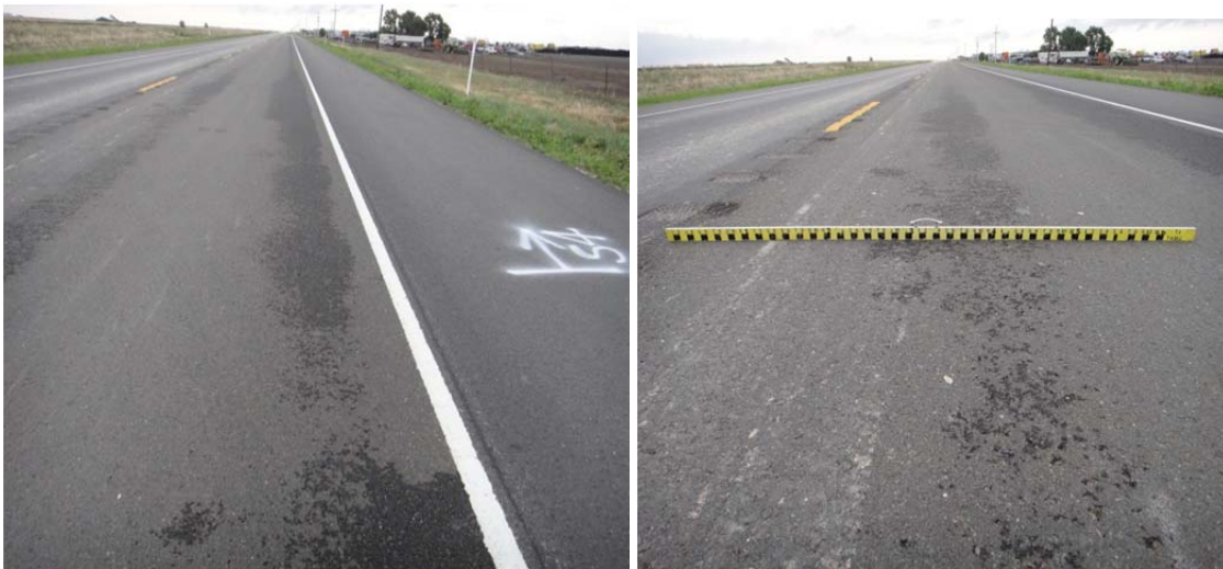
Figure 58. Field Survey of SH 15 Test Sections.
