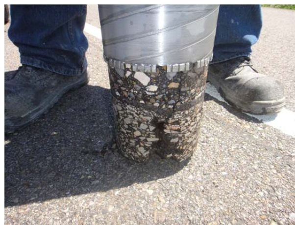
Figure 65. A Typical Core Indicating Reflective Cracking on US62.
