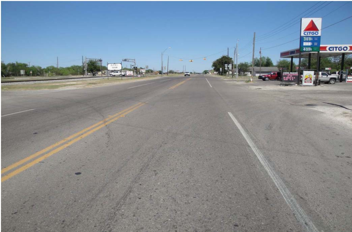
Figure 48. Overview of the SH359 Test Section.
