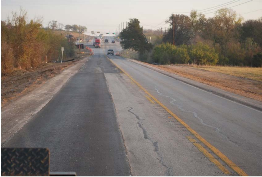
Figure 53. Patching Area prior to Paving at the North End of the Test Section.
