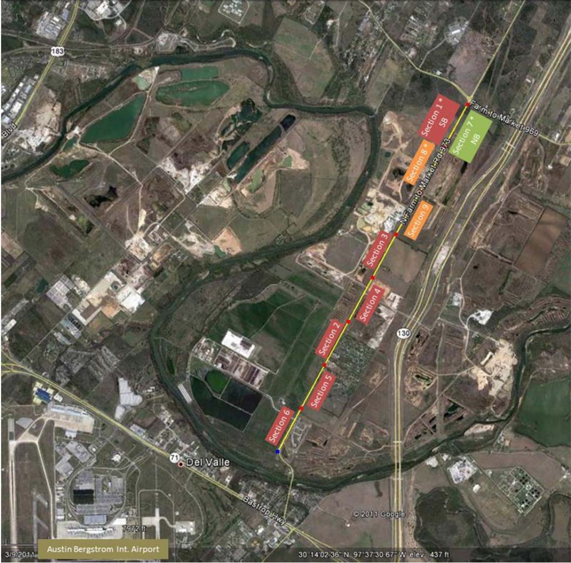
Figure 50. Project Limit with Satellite View.
