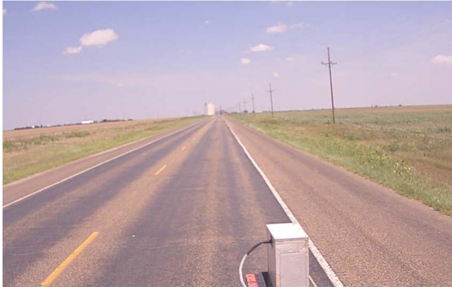
Figure 57. Existing Pavement Condition of SH15 Test Sections.
