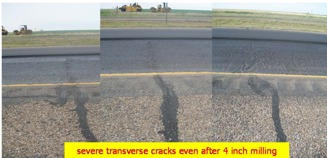
Figure 38. Existing Pavement Conditions of IH40 after Milling.
