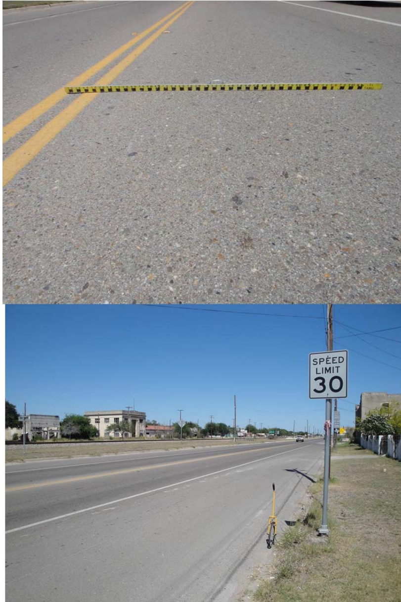
Figure 49. No Crack, No Rutting in the SH359 Test Section, as of 12/20/2012.
