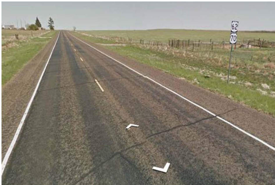
Figure 60. Existing Pavement Conditions of US62 Test Sections.
