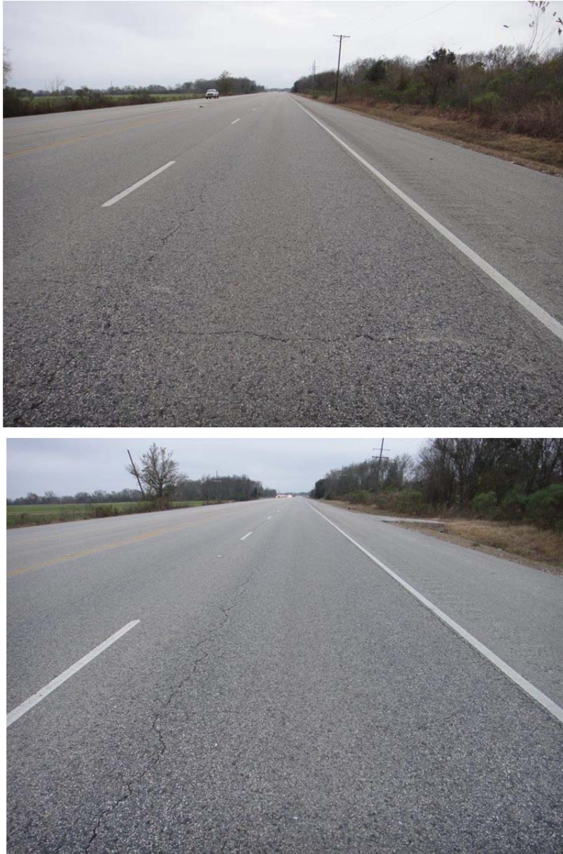
Figure 46. Pavement Condition of the RAP/RAS Test Section on SH146, Houston on December 18, 2014.
